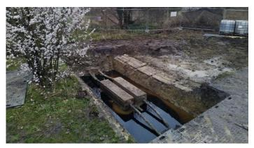
of them unfortunately had sprung a leak in a joint which was seeping insulating oil into the soil. Despite the disruption of the excavation, and the sea of mud caused by removing the contaminated soil during yet more wet weather, by the summer there was little sign of the destruction caused. Nature is good at healing.
