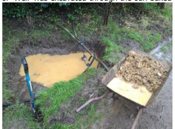
hardened earth in the chosen area. During the wet winter it was enlarged and a lot easier to dig! A small pump with an automatic float switch was installed, and an inch bore hose attached.
